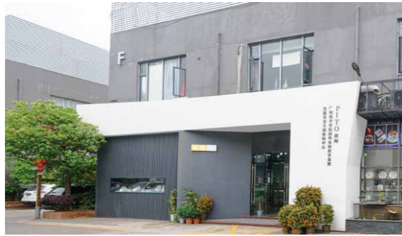
GBI / Catering Products Experience Center / Consulate kitchen
